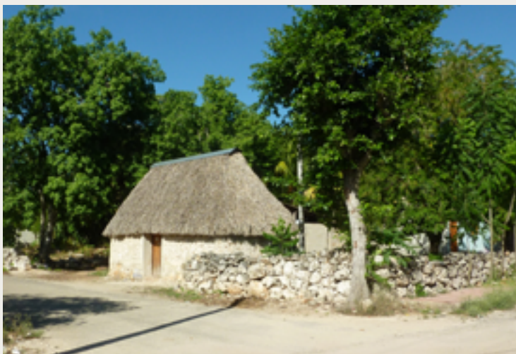
Figure 14: Mayan house with lime-stone masonry walls. Photo by BAP
