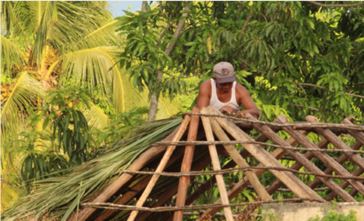
Figure 7: Palm placement for the roof. Photo by FJMS*
