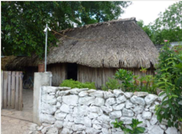
Figure 15: Mayan house with bajareque walls. Photo by BAP
