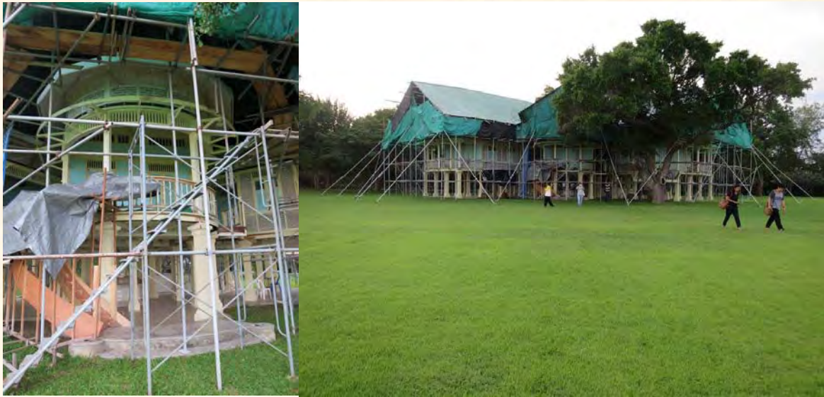
8-9) Chao Praya Ramaraghave Villa renovation project of Mrigadayavan Palace Foundation / Photo: Pongkwan L.
