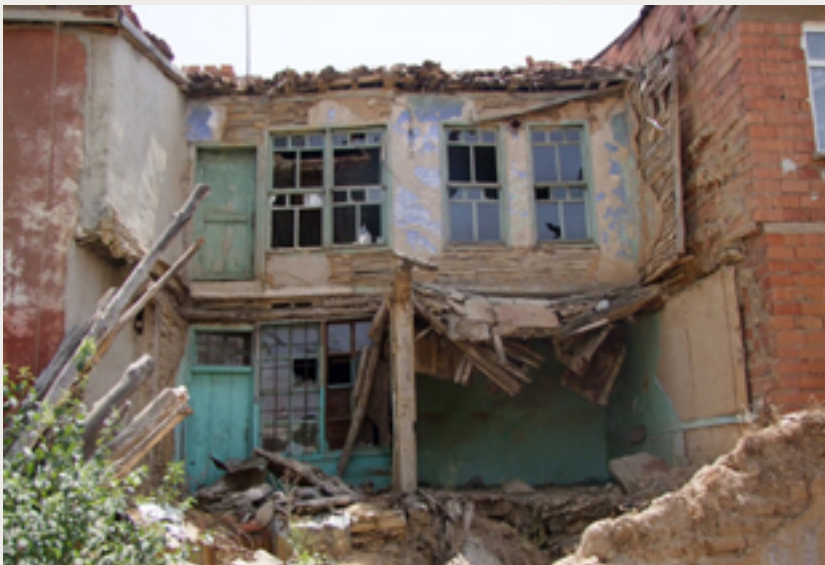
Figure 7. The current state of the foreign houses (Arslantaş, 2020)
