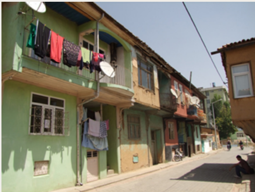
Figure 5. Foreign houses in Ilgın (CERAY Architecture, 2010)
