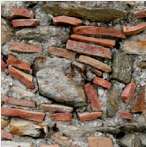
Figure 3. Wall enclosures (Alcindor)
