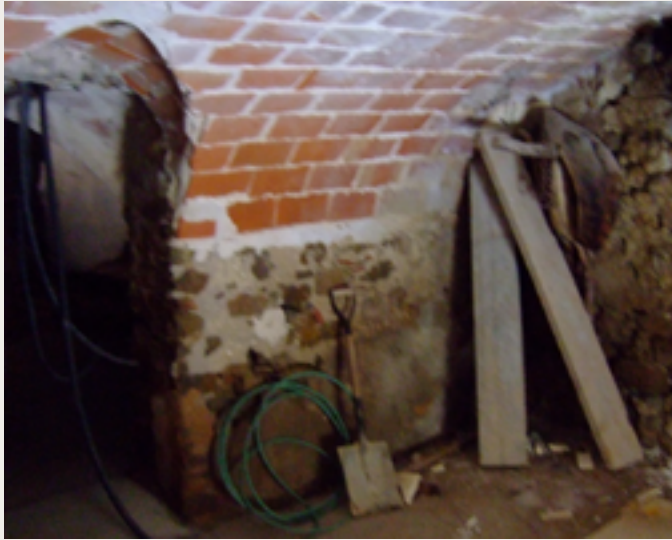
Figure 1. Examples of the houses before and during the intervention (Empordanet) (Alcindor)
