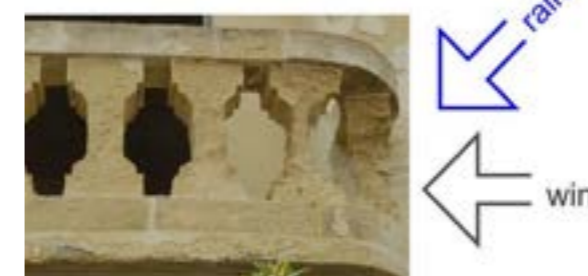
Fig.2 Stone as a balcony surround. At first sight, it could be decoration but in fact it is destruction. The left baluster is untouched but the right one has been ruined by rain. Is it the wrong choice of material, or merely the wrong side of the facade? Perhaps both. © The author
