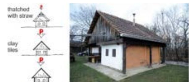
Fig.7 The walls normally carry the roof construction, together with the roofing material. Original roofing material was straw: it needs very light construction. When fired clay tiles arrived, because of less maintenance and greater safety, the construction had to be stronger, bigger and heavier. Problems with earthen walls began. An outer, wooden construction from the foundation to the top seems to be reasonable. © The author
