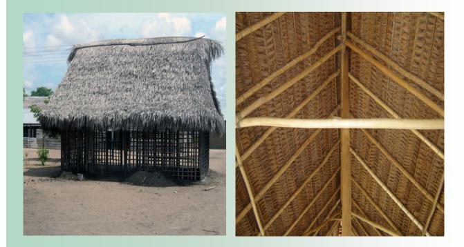
The roof structure was planned solution and venting of hot air from inside, through openings in the corners of the cover and the protection of the earthen walls with pronounced eaves.
