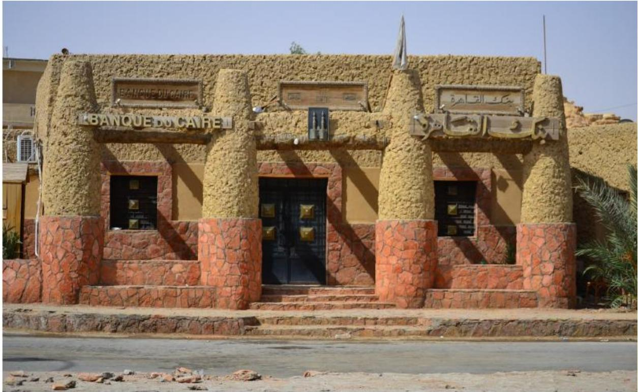
Local bank branch designed and constructed by The Siwa Sustainable Development Initiative with earth vernacular building technology in the Siwa oasis using Karshif. According to the designer, the building passed safety and security bank tests in 2008. It is a trial to revitalize traditional vernacular building technique that is about to vanish
