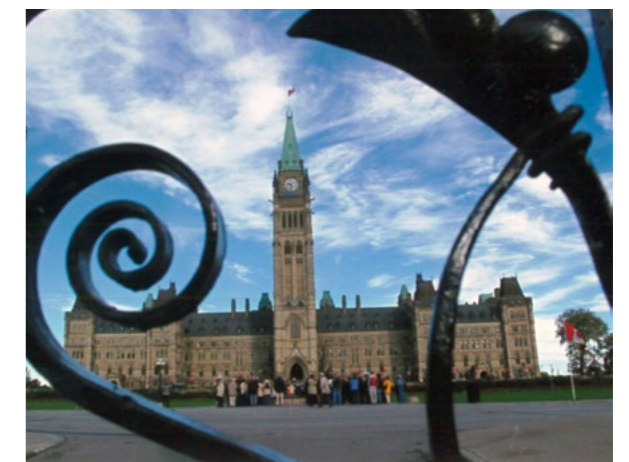
Restoration of the historical fences, Vaux Walls & North Wall. Masonry maintenance of West, East & Centre Block, restoration of some interior's rooms © María Inés Subercaseaux
