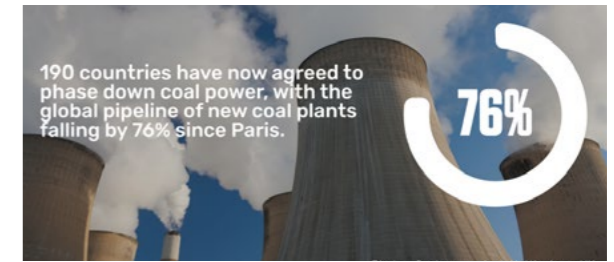
Coal Power Plant in Nottingham, UK. Source: E3G
