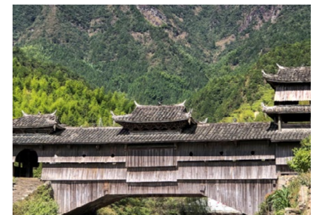
Rulong Bridge: China's oldest woven-arch timber bridge constructed during the Ming dynasty in 1625 and renovated between 1821 and 1859 during the Qing dynasty. © Ronald G. Knapp, 2019.
