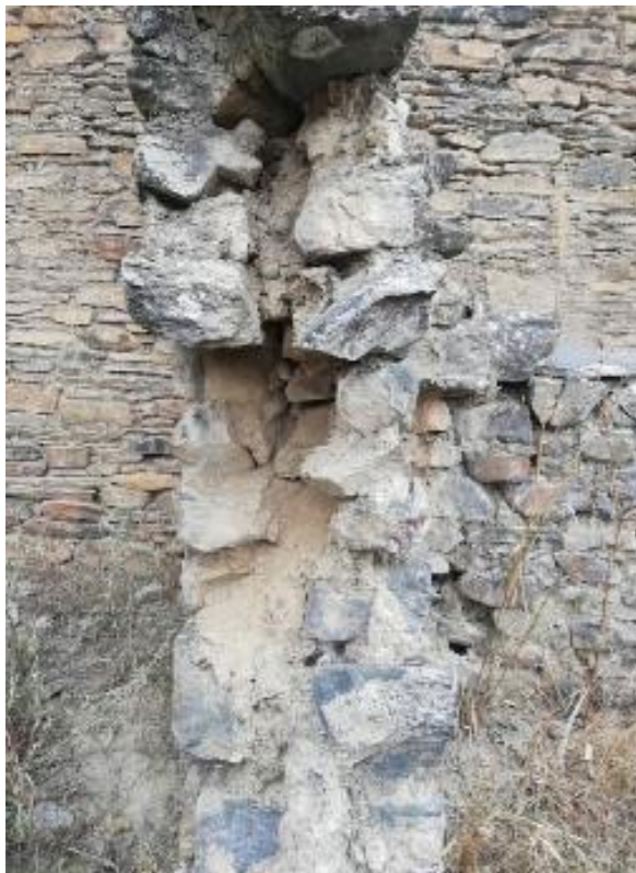
Fig.3 ROOM WALL SECTION WHERE THE COMPOUND WALL IS OBSERVED. © The author
