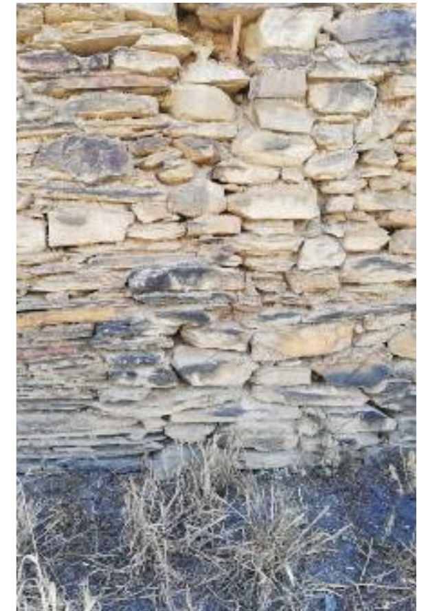
Fig.4 DETAIL OF THE RETAINING WALL SHOWS THE LEVELING AND LOADING SECTIONS. © The author
