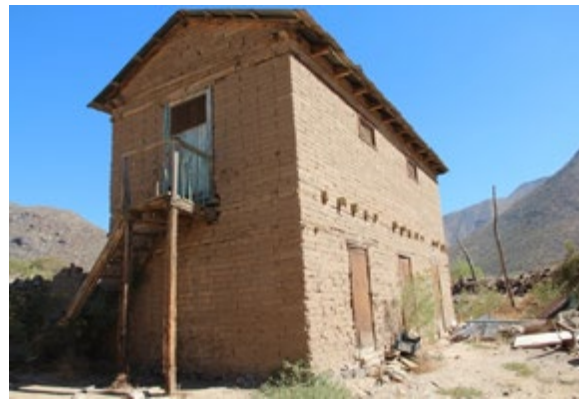
Fig.9 Rural two-floor construction in Monte Patria. Case with mass and horizontal ladders. State after the earthquake of 2015 © Amanda Rivera, 2016
