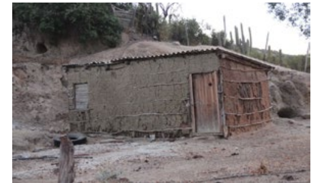
Fig.2 Quincha of the “Norte Chico” with medium size branches as structure. © Amanda Rivera, 2016
