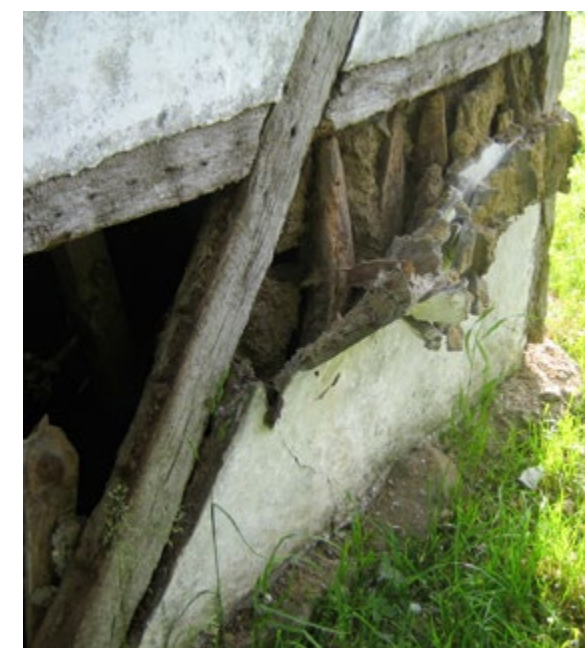
Fig.4 Chicken wire and cement made a false impression of a sound construction. Behind the surface the wood and daub were in poor condition. © The author
