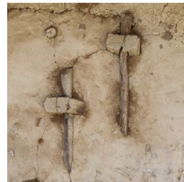
Fig.6 Trabas: Wooden pieces to join perpendicular walls in the town of Cogotí 18 © Amanda Rivera, 2016
