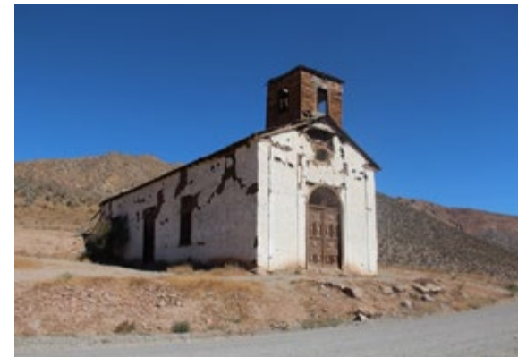
Fig.10 Rural abandoned church in Río Hurtado. Case with mass and horizontal ladders. State after the earthquake of 2015 © Amanda Rivera, 2016
