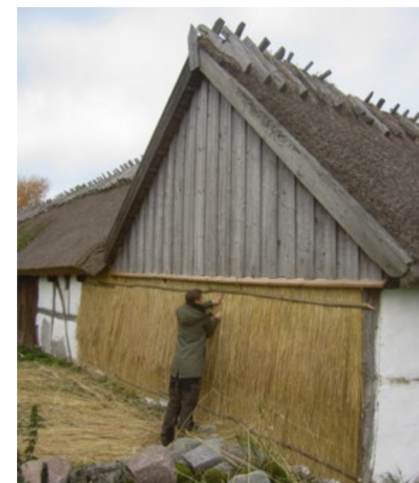
Fig.8 Historic sources gave us information of one traditional way of making the maintenance intervals longer. It is called “byrning” and is made by putting rye straw on the walls only fastened with hazel rods nailed to the frame. © The author
