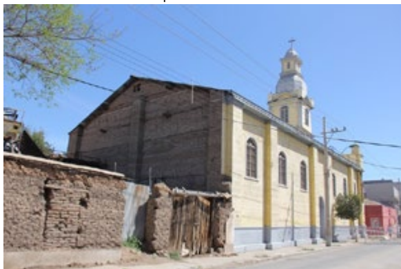
Fig.8 Corazón de María church in Ovalle. Case with mass, counterforts and horizontal ladders. State after the earthquake of 2015 © Amanda Rivera, 2015
