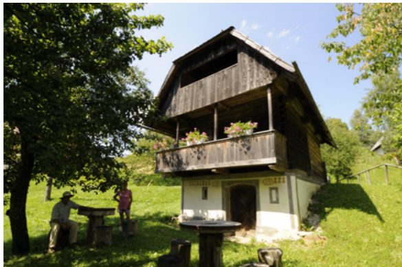
Fig.4a Granary on the Mountain Pohorje has cellar, living room and attic © The author
