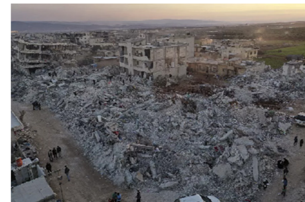
People walk past collapsed buildings following a devastating earthquake in the town of Jinderis, Aleppo province, Syria, Thursday, Feb. 9, 2023. © Ghaith Alsayed/© 2023 The AP
