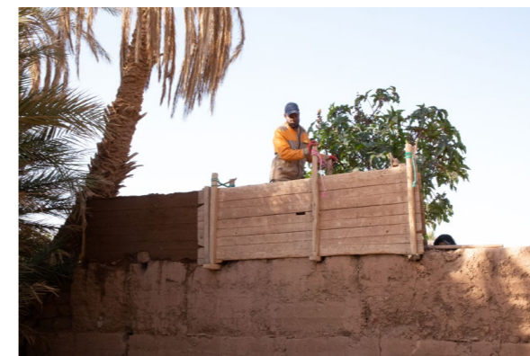
Fig.6 Construction of rammed earth wall in Ksar Ouled Driss, ©ArCHIAM 2023.
