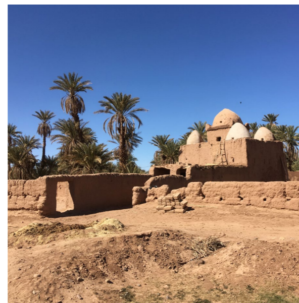
Fig.5 South-east view of the Marabout of Sidi Abdellah Khalifa in Ksar Ouled Youssef, ©ArCHIAM 2019.
