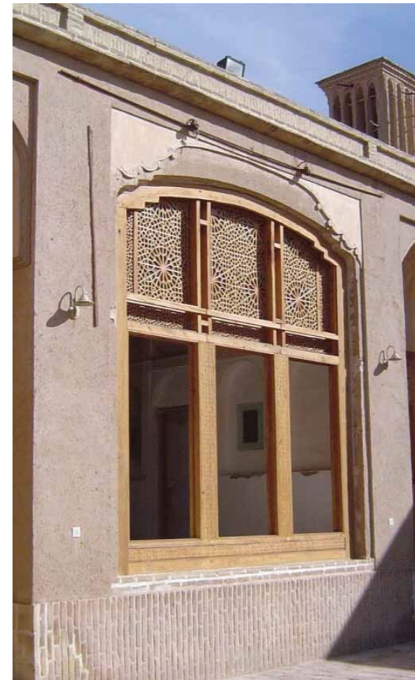
Fig.5 A sash-window in Yazd. Source: Photograph by the author
