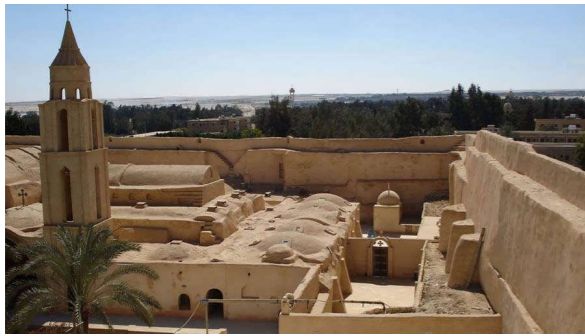
Figure 8 Boundary, Baramous monastery, Wadi El-Natrun, 9th c. In addition of the inner surrounding corridor for the guard monk there is a number of openings to watch while protecting himself.
