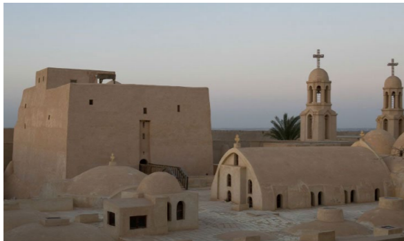
Figure 9 The keep, Baramous monastery, Wadi El-Natrun, 9th c. From the roof the church. On this image appears the bridge to access into the keep. The existing roof of the church is not the original one, which was probably constructed with timber. Using pointed vaults and domes began in churches with introducing the Islamic culture.
