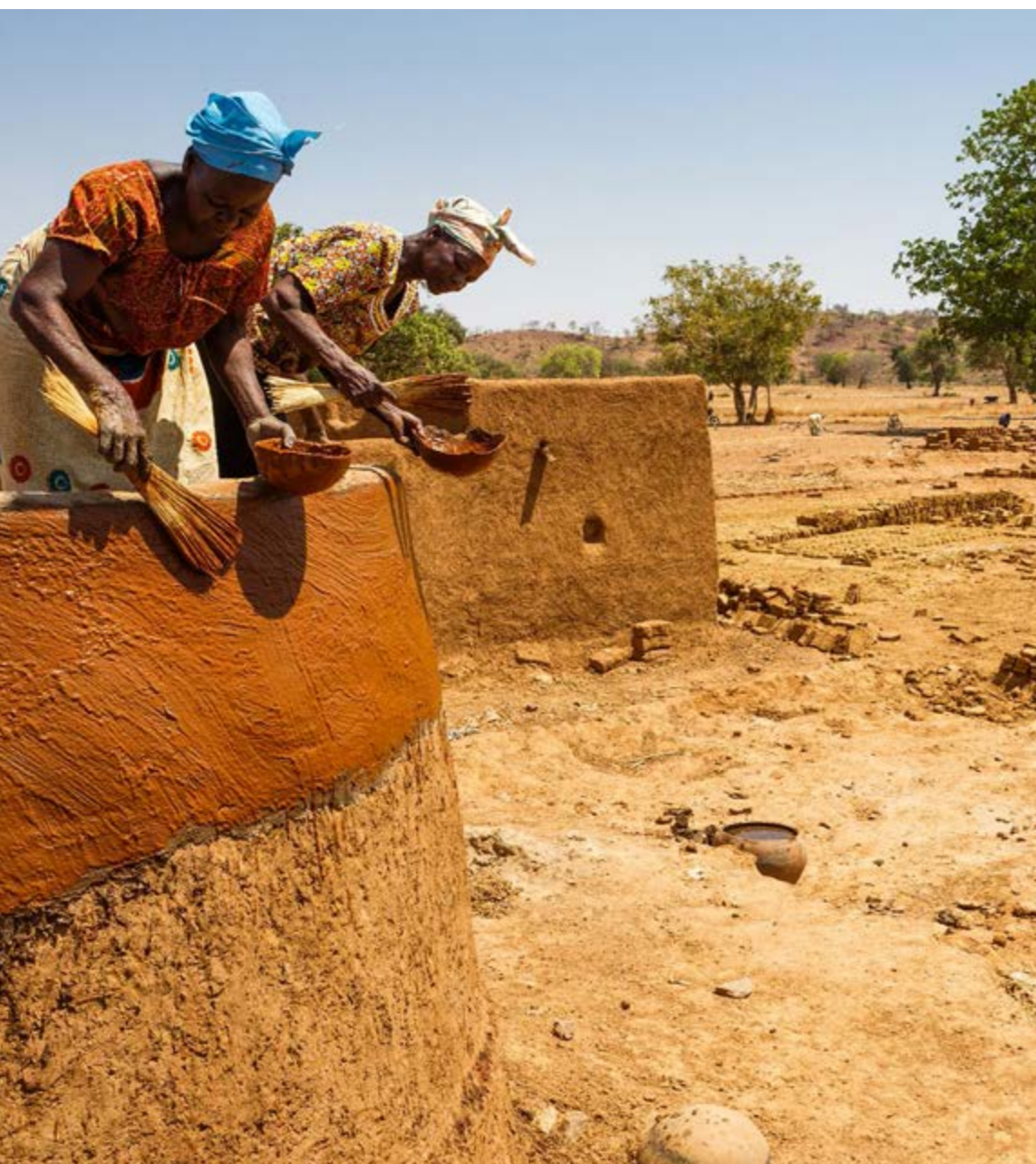
Kassen a habitat. Women working on their houses. ©Burkina Faso Architecture, Culture and Cooperation
