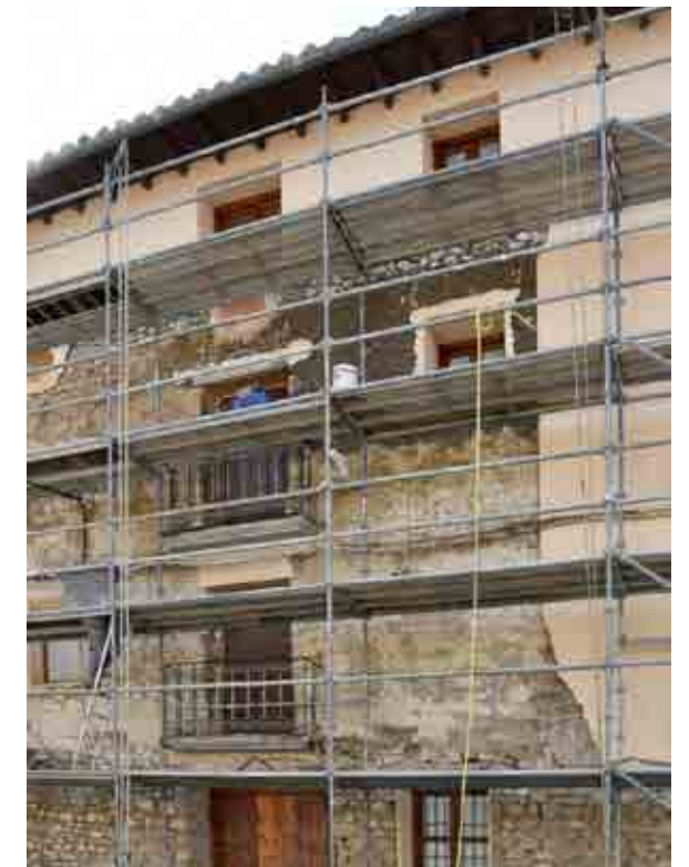
Fig. 2 Intervention in a historic building in Forcall (Castellón), using industrial materials such as cement mortar. © The author
